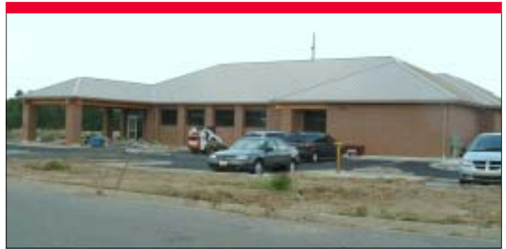
First Dayton Cancer Care under construction.
